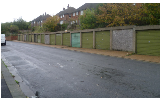
View looking North into the site from Buckley Close
